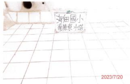
(南棟東側)水塔清洗後
