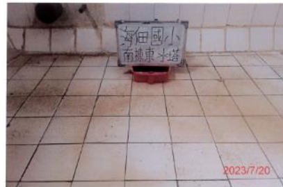
(南棟東側)水塔清洗前
