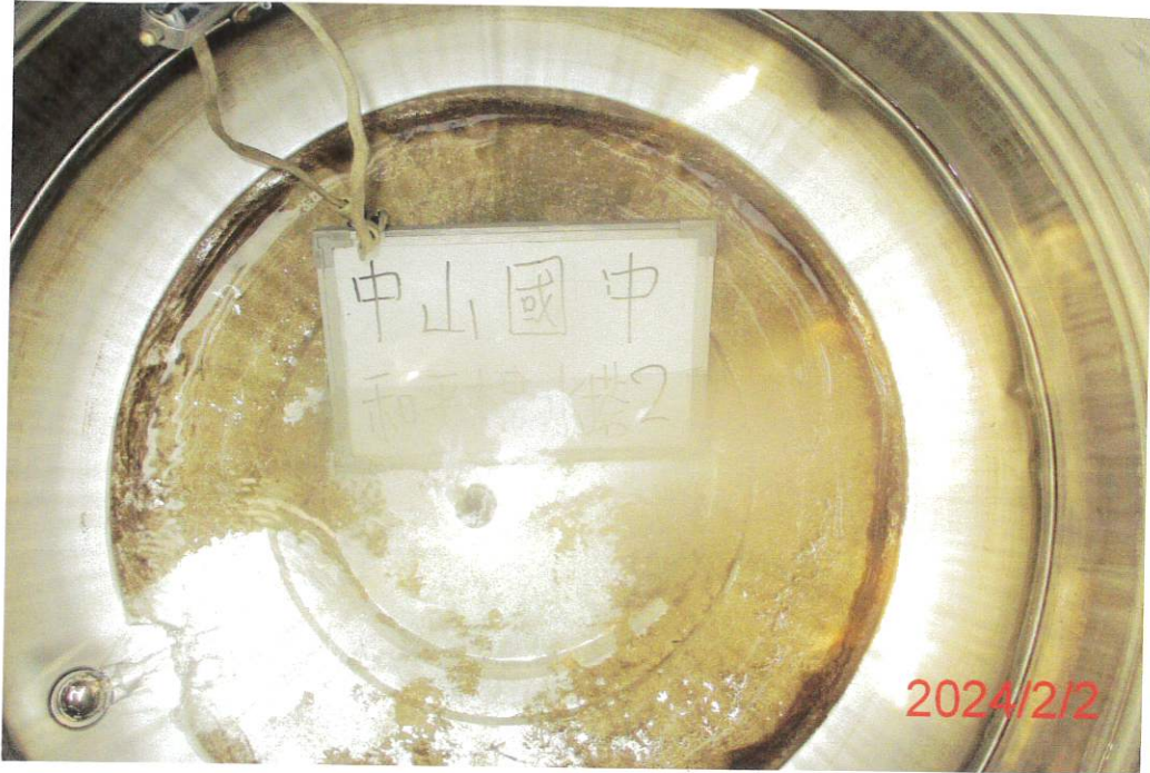
(和平樓-2)水塔清洗前
