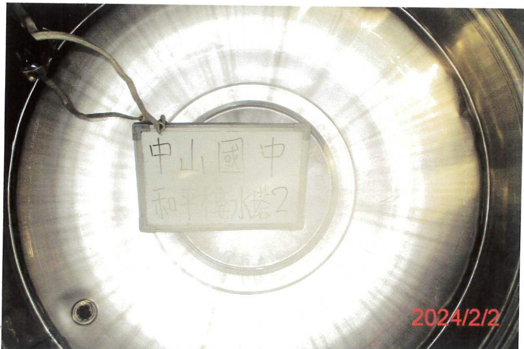
(和平樓-2)水塔清洗後
