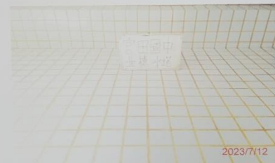
(北棟)水塔清洗後
