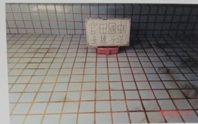
(北棟)水塔清洗前
