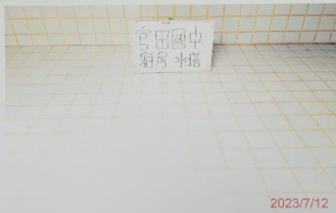
(廚房)水塔清洗後
