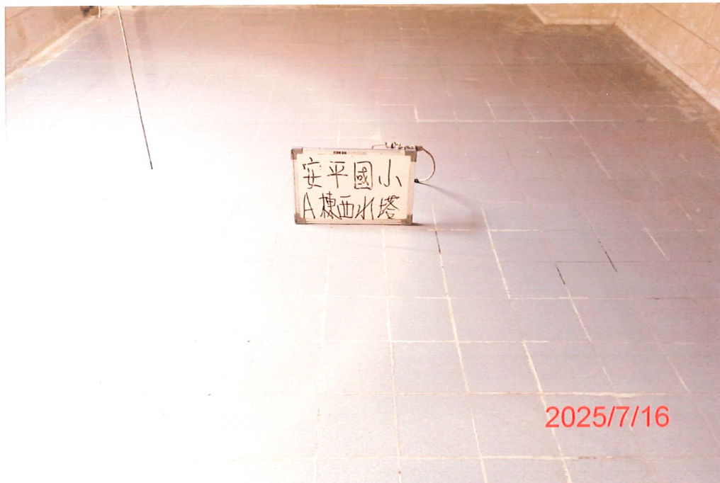
(A棟西)水塔清洗後
