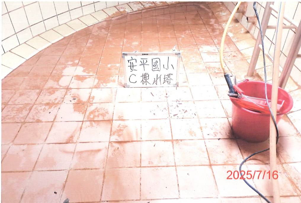
(C棟)水塔清洗前
