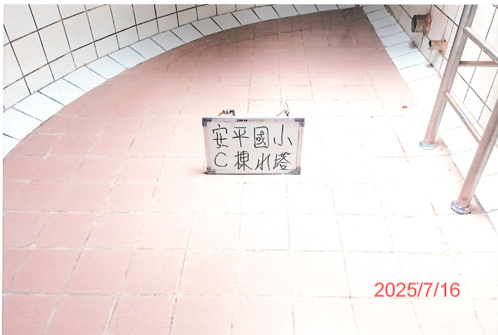
(C棟)水塔清洗後
