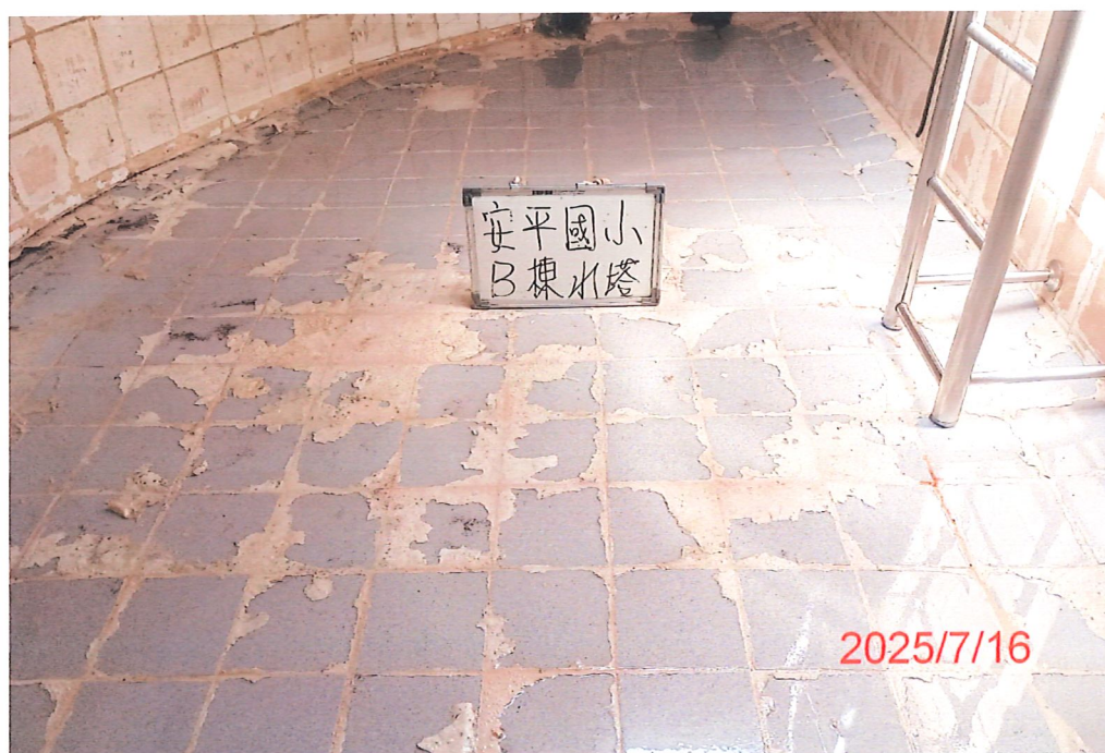
(B棟)水塔清洗後
