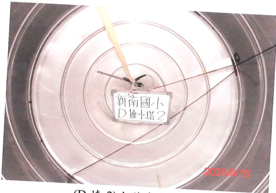
(D棟-2)水塔清洗後
