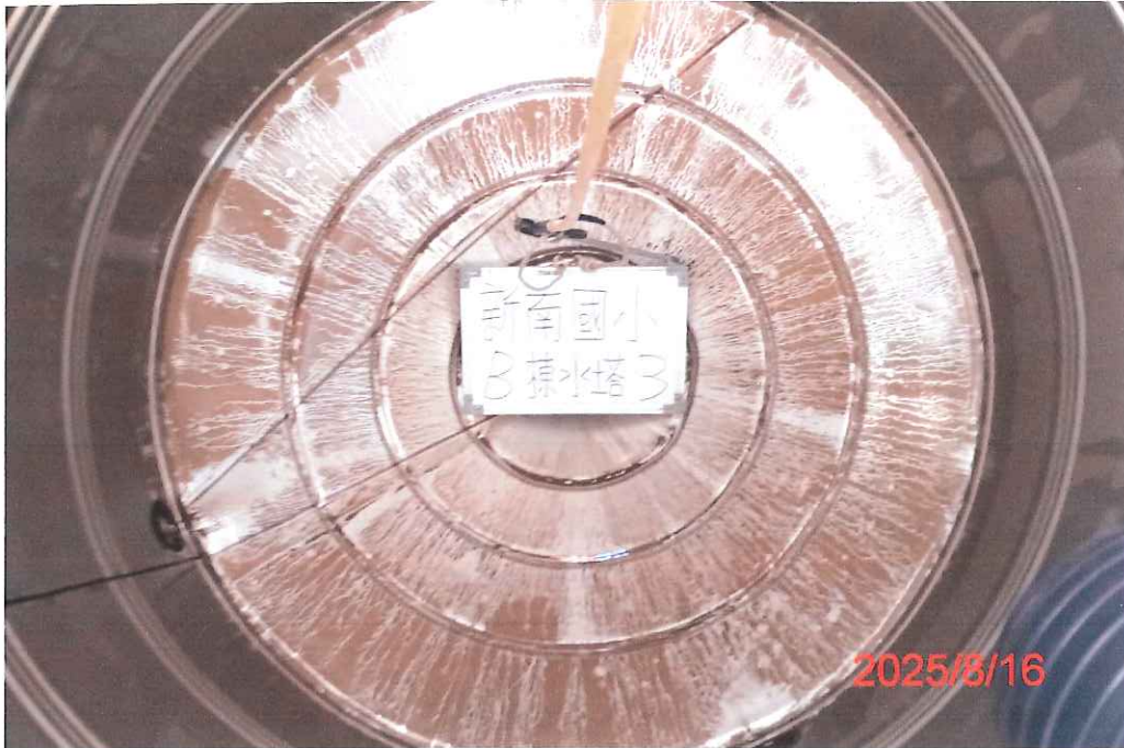
(B棟-3)水塔清洗前
