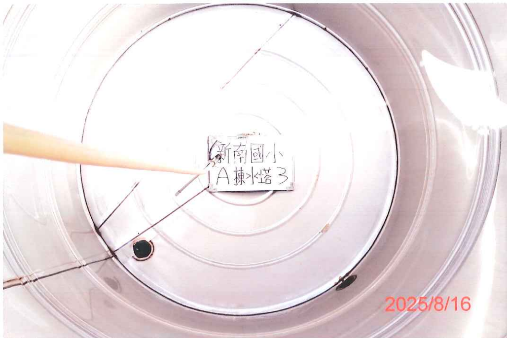
(A棟-3)水塔清洗後
