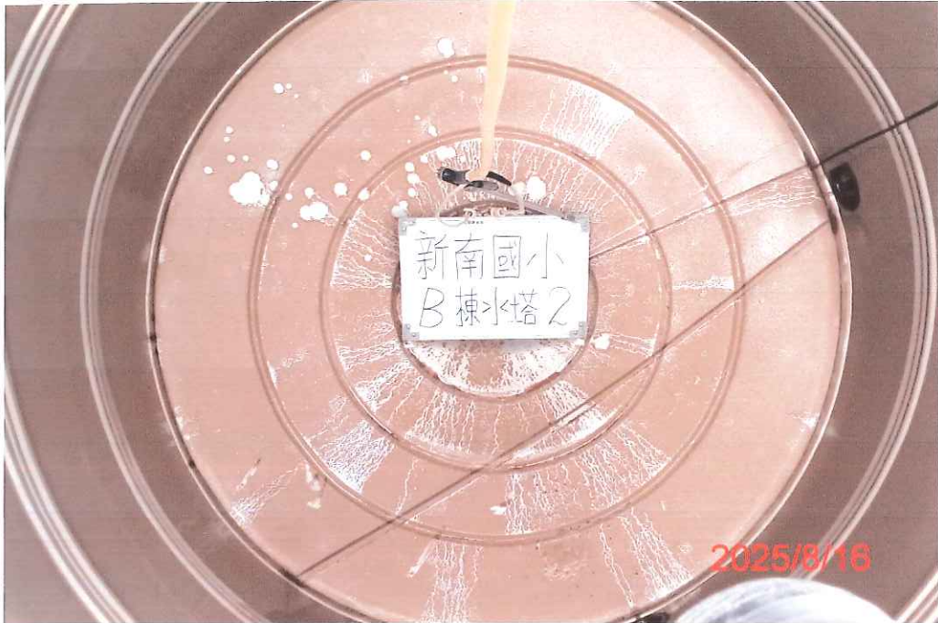
(B棟-2)水塔清洗前
