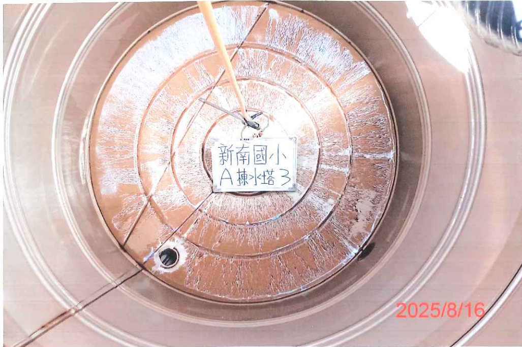
(A棟-3)水塔清洗前
