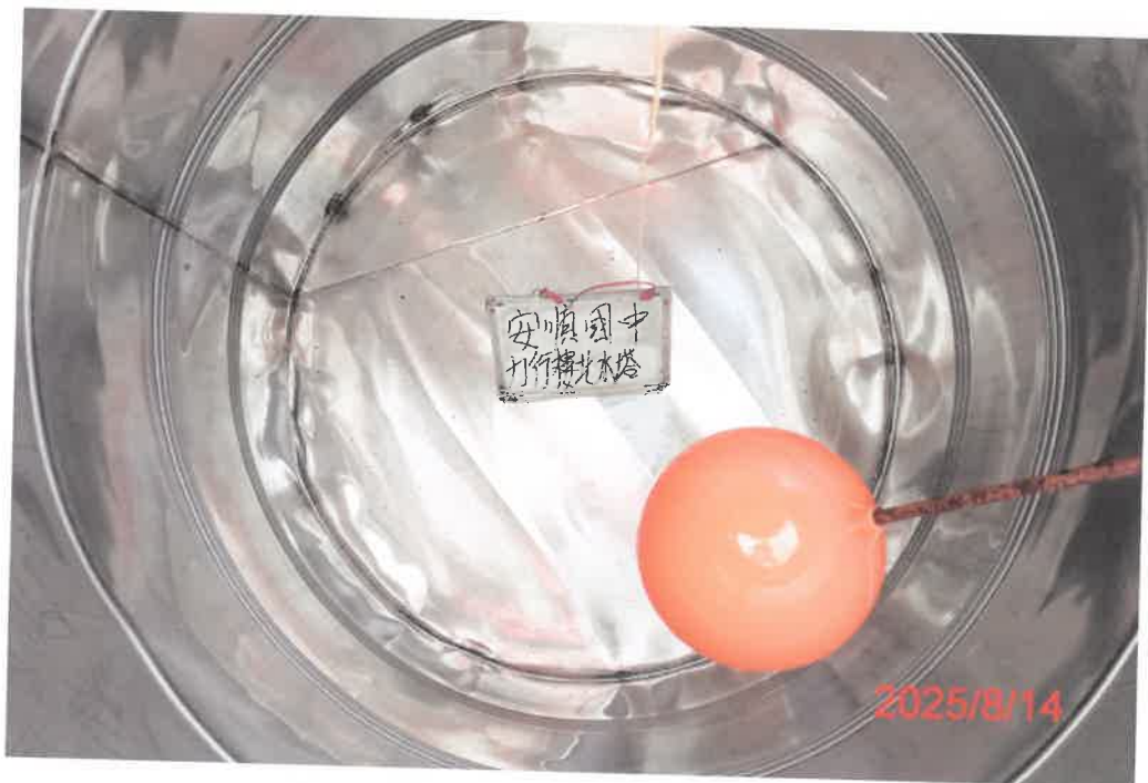
(力行樓北-1)水塔清洗後
