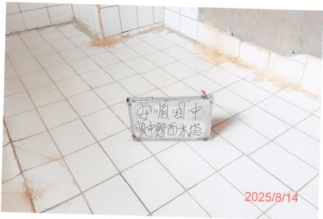
(順中館西)水塔清洗後
