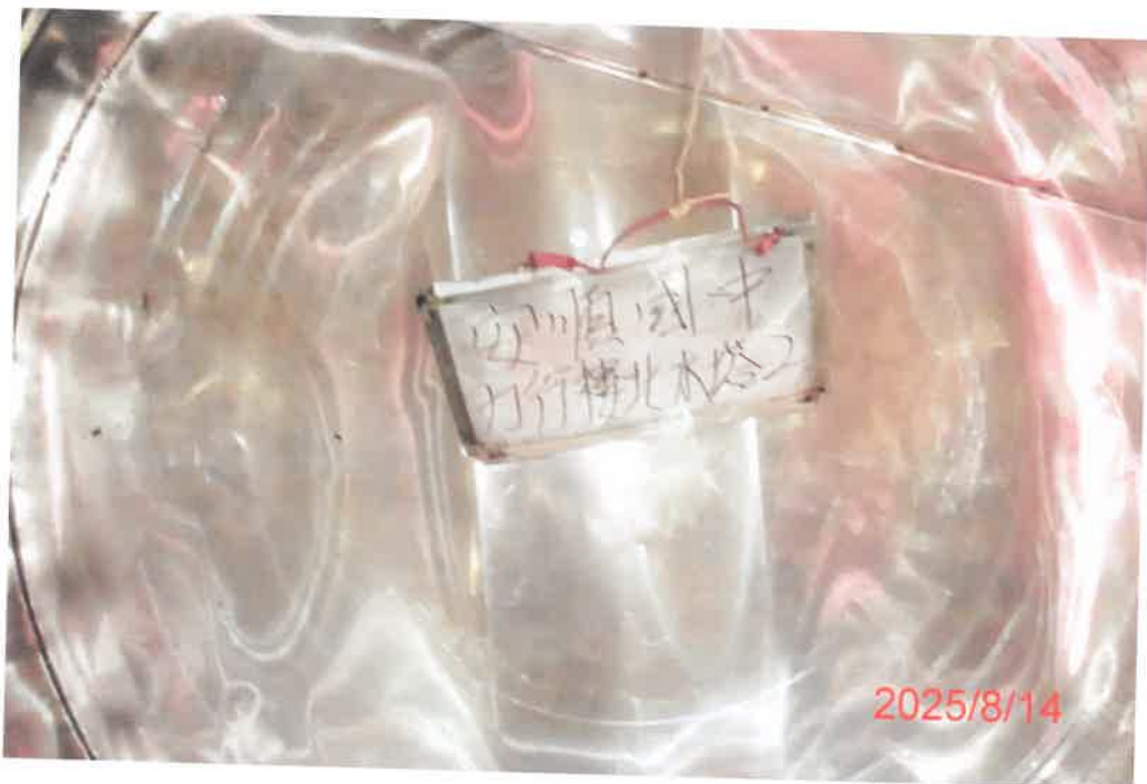
(力行樓北-2)水塔清洗後
