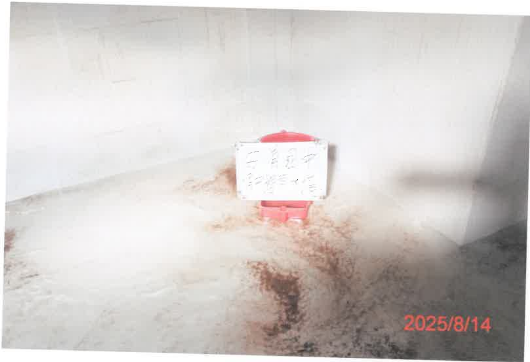
(順中館東)水塔清洗前
