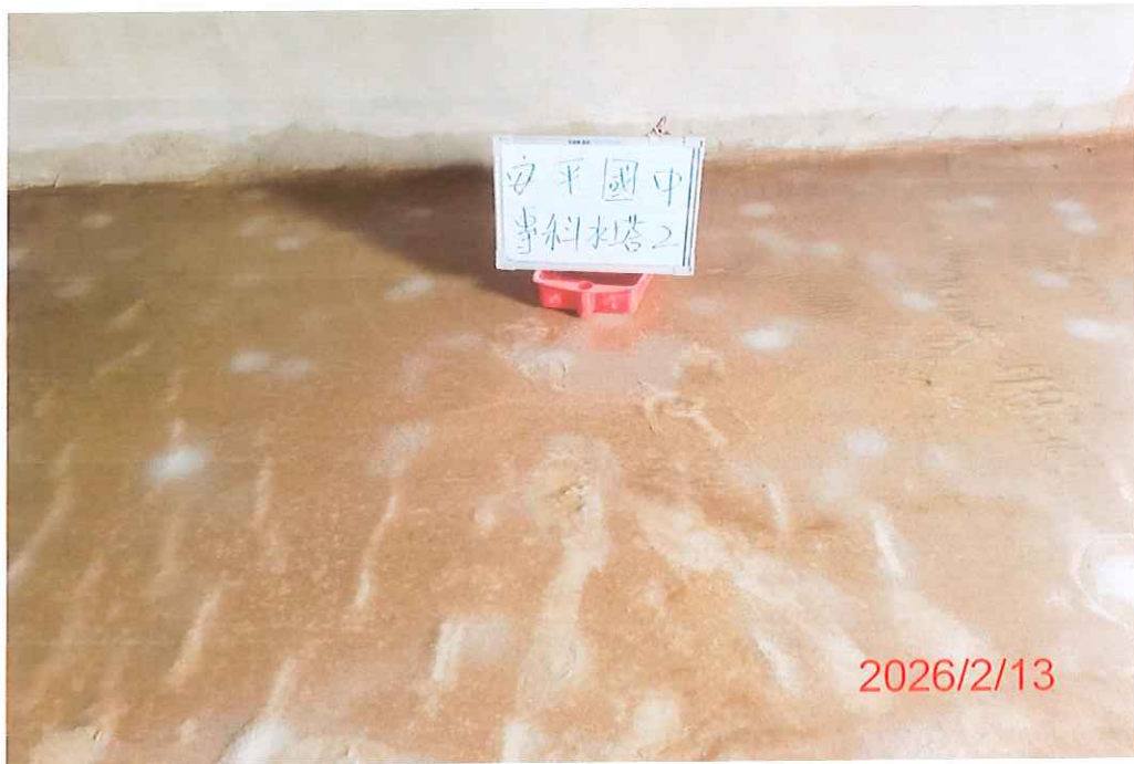
(專科大樓-2)水塔清洗前
