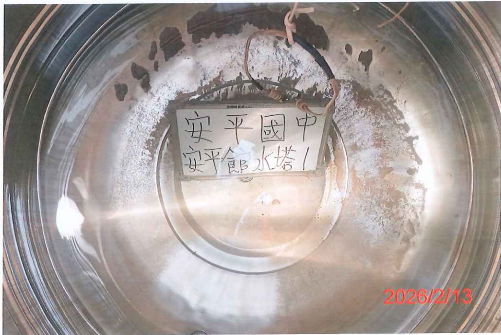
(安平館-1)水塔清洗前
