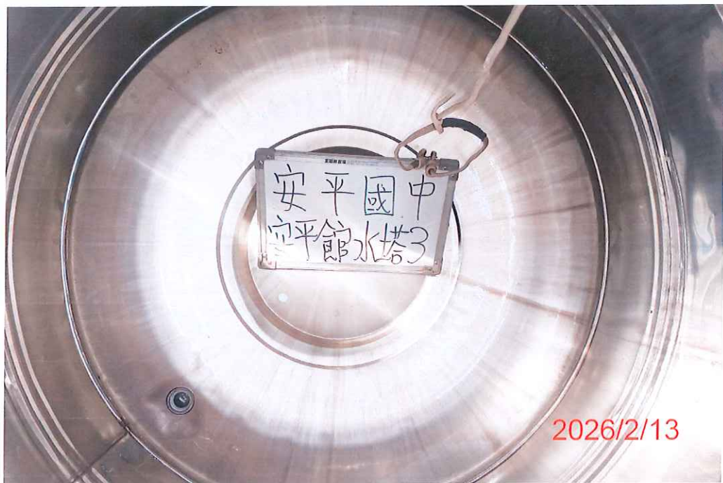
(安平館-3)水塔清洗後
