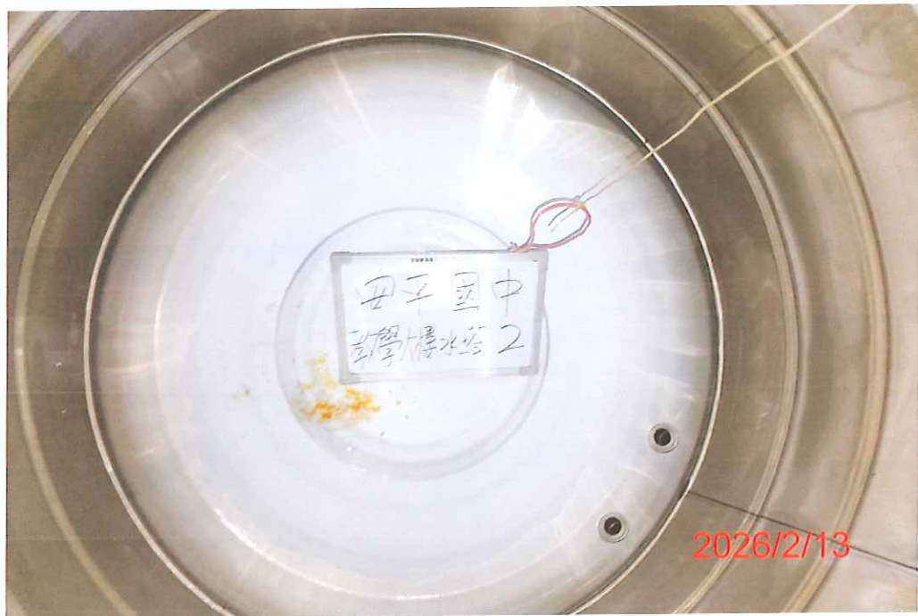
(教學大樓-2)水塔清洗後
