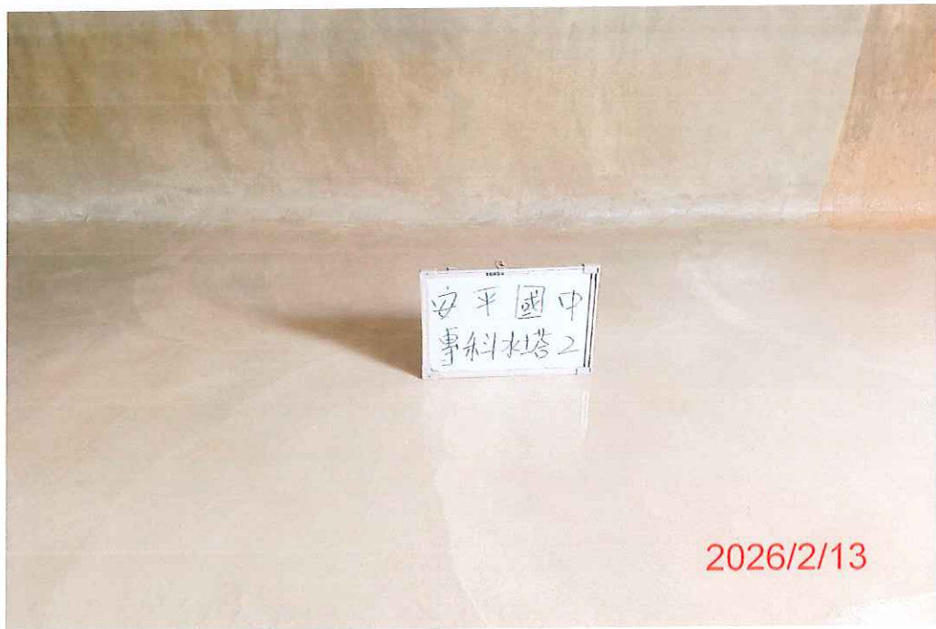
(專科大樓-2)水塔清洗後
