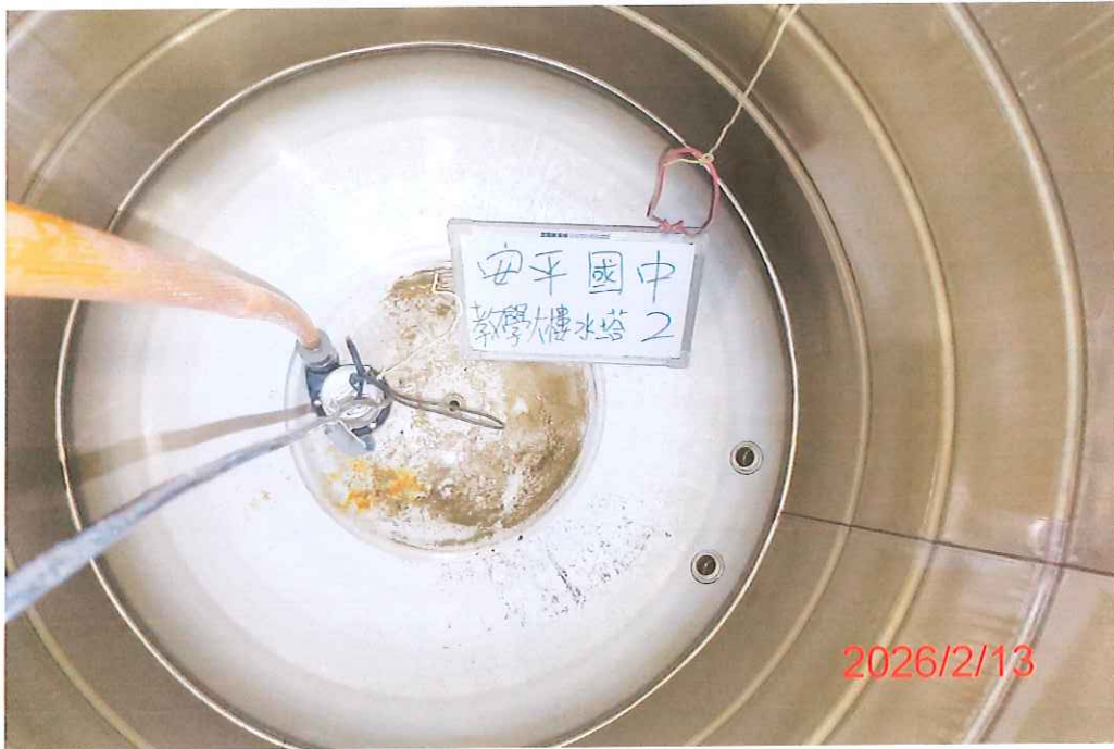
(教學大樓-2)水塔清洗前
