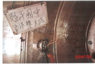
(勤學樓)水塔清洗前
