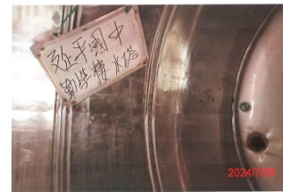
(勤學樓)水塔清洗後
