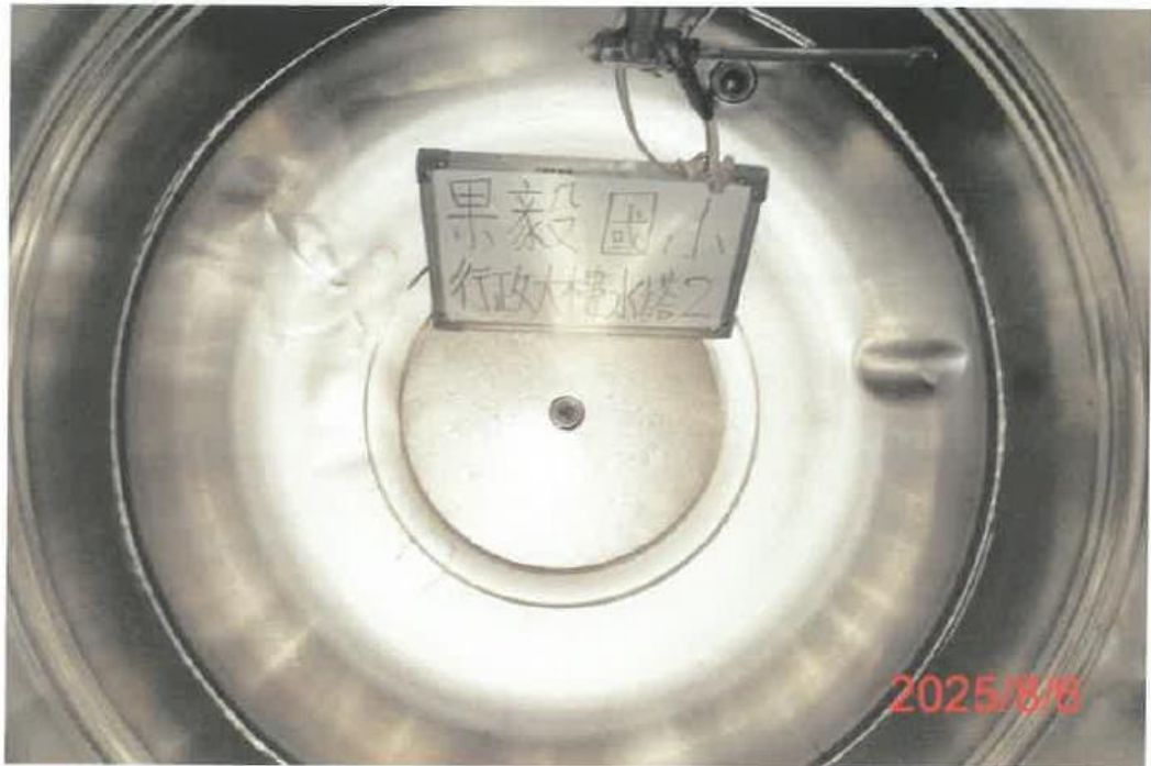
(行政大樓-2)水塔清洗前
