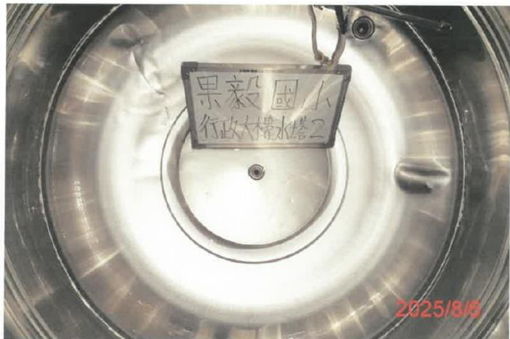
(行政大樓-2)水塔清洗後
