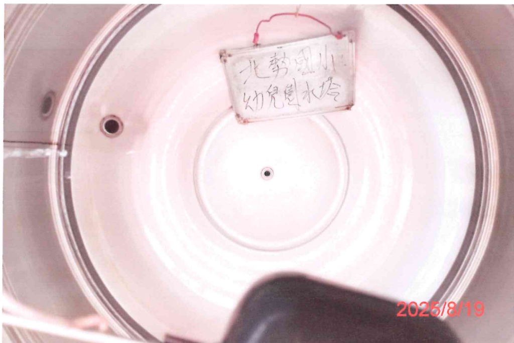
(幼兒園)水塔清洗後
