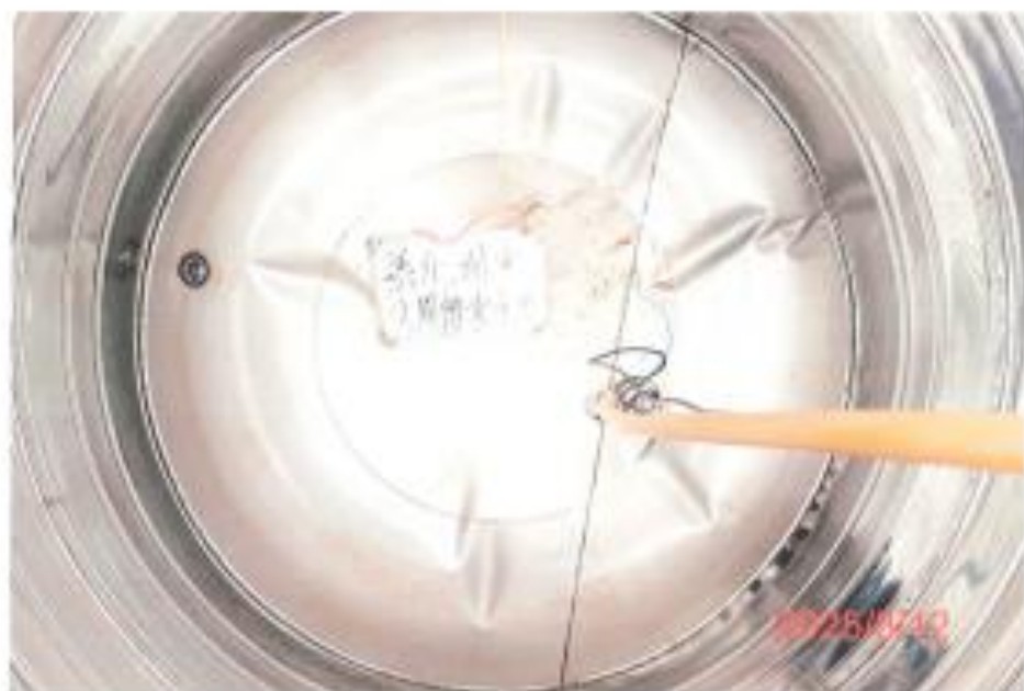
(文開樓東)水塔清洗前
