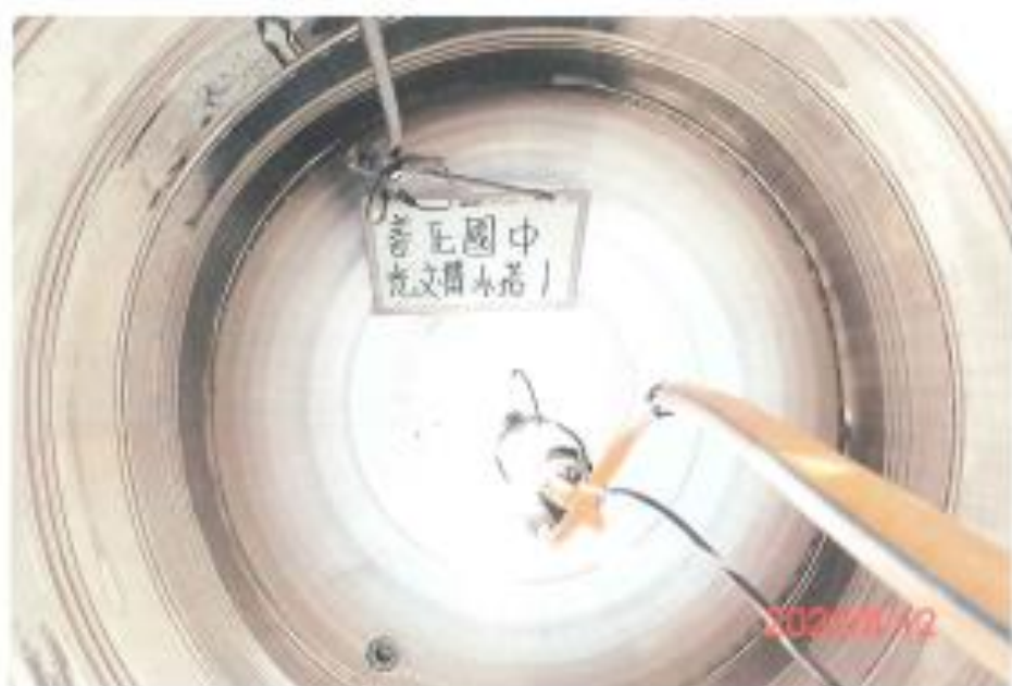
(光文樓-1)水塔清洗前
