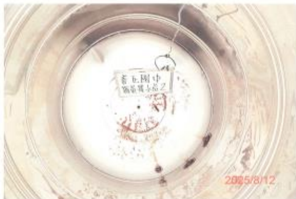
(斯菴樓-2)水塔清洗前
