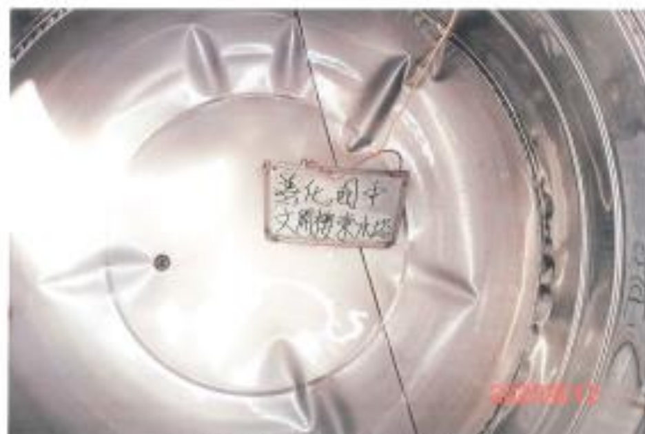
(文開樓東)水塔清洗後
