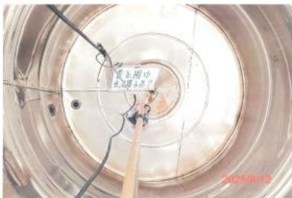
(光文樓-2)水塔清洗前
