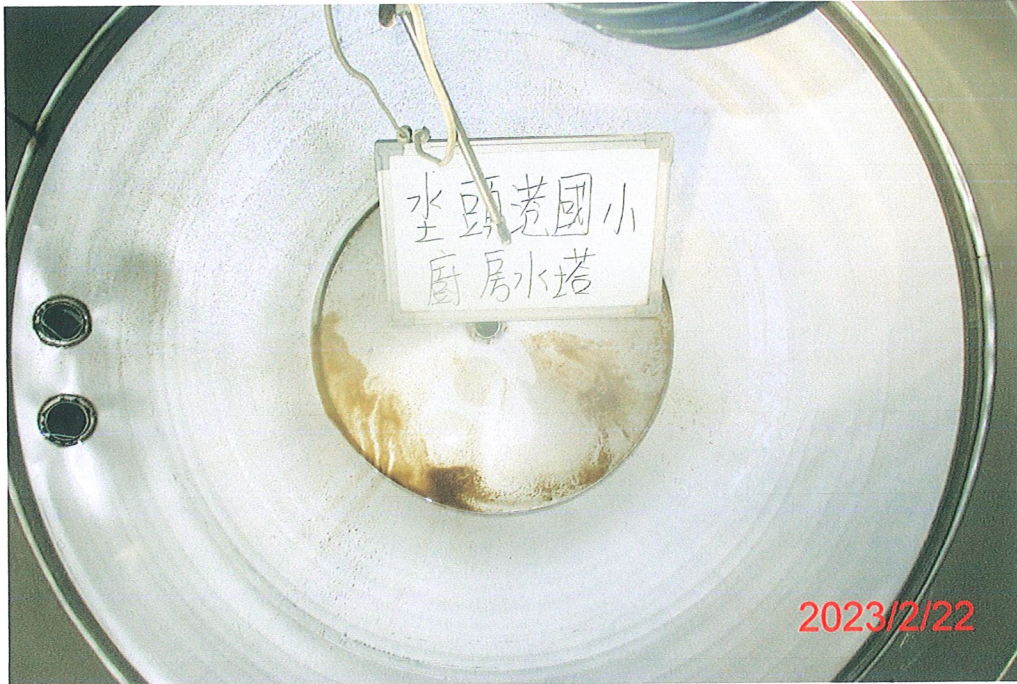
(廚房)水塔清洗前
