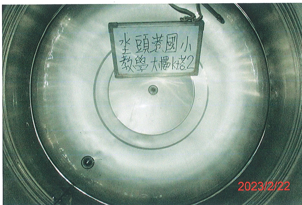
(教學大樓-2)水塔清洗後
