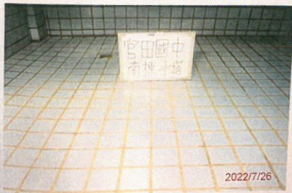
(南棟)水塔清洗後
