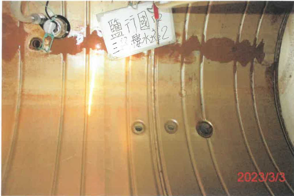
(三民樓-2)水塔清洗前
