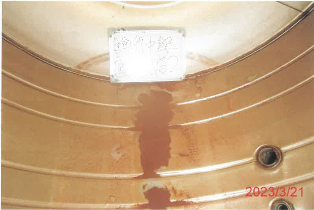
(鹽行樓-2)水塔清洗前
