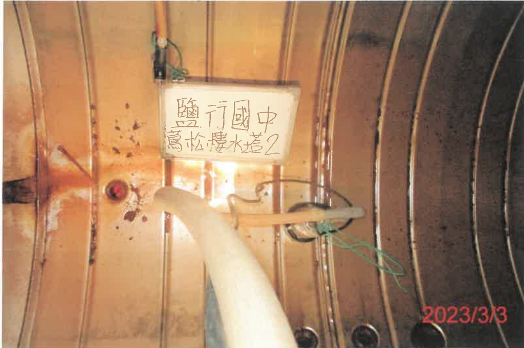
(蔦松樓-2)水塔清洗前
