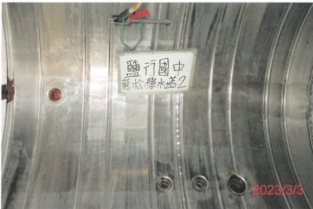
(蔦松樓-2)水塔清洗後
