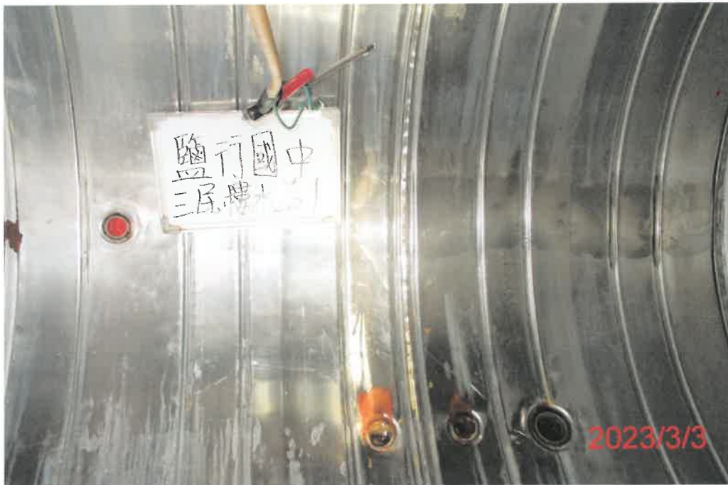
(三民樓-1)水塔清洗後
