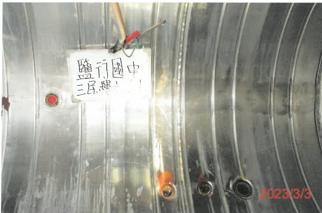
(三民樓-1)水塔清洗後
