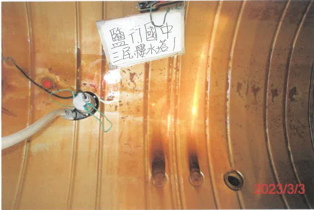
(三民樓-1)水塔清洗前
