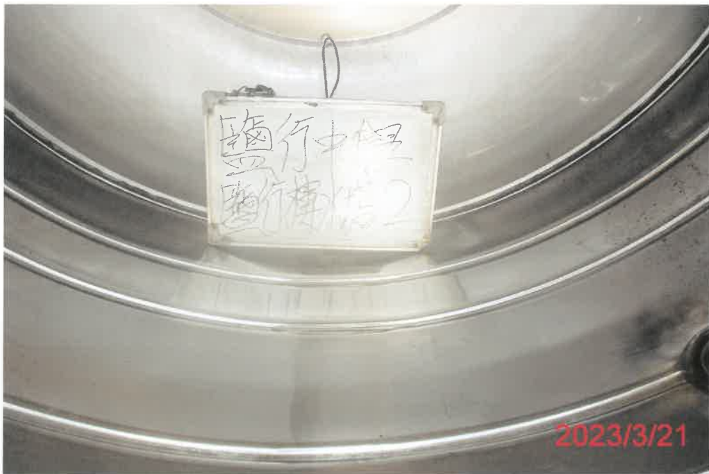
(鹽行樓-2)水塔清洗後
