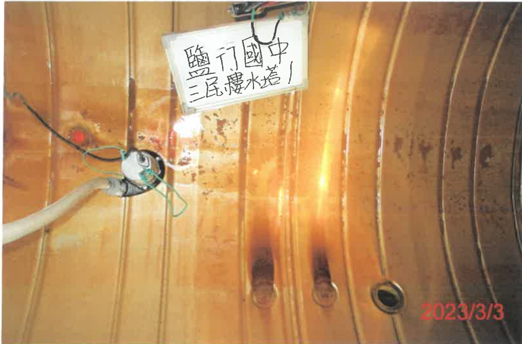
(三民樓-1)水塔清洗前
